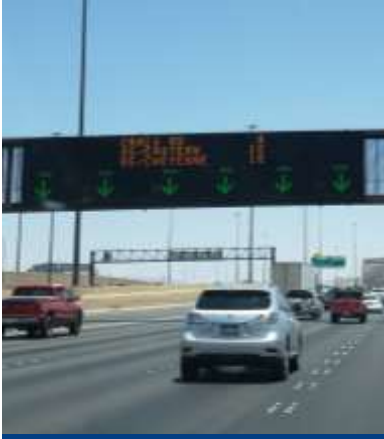
US-95 Integrated Safety Technology Corridor
